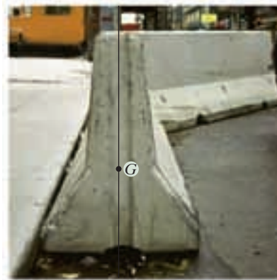
In order to determine the force required to tip over this concrete barrier it is first necessary to determine the location of its center of gravity G . Due to symmetry, G will lie on the vertical axis of symmetry. (© Russell C. Hibbeler)
